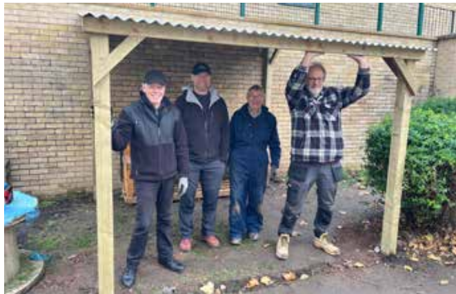
Men in sheds members at Lyde Green Primary School
