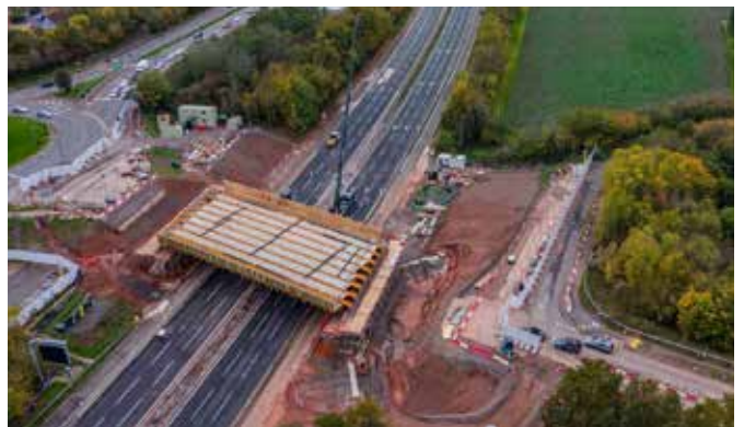
The bridge with all beams fitted. Picture: National Highways.
