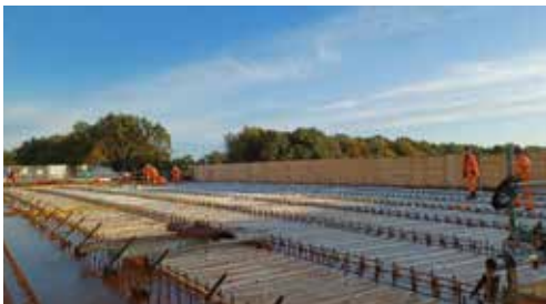
Workers on the deck of the bridge. Picture: National Highways.
