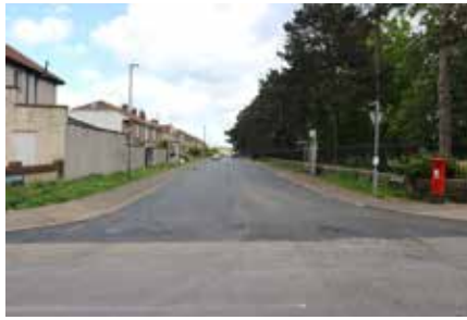
South View is being resurfaced
