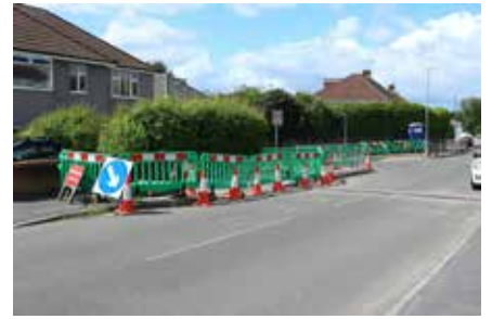
A zebra crossing is being installed on Four Acre Road
