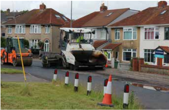
Resurfacing work in Northcote Road
