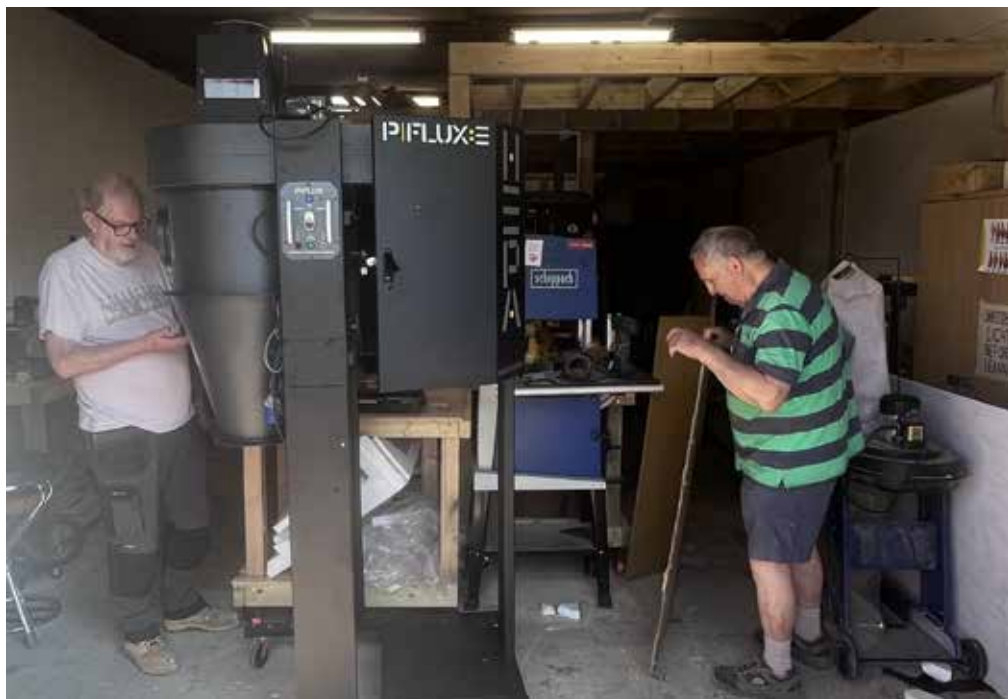
Fitting the dust extractor
